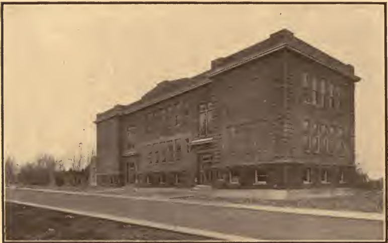
WEST FRANKFORT HIGH SCHOOL
